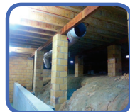
Sub Floor Ventilation
